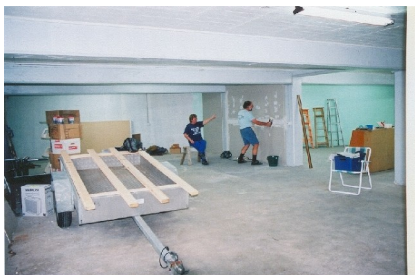
Gib board being plastered
